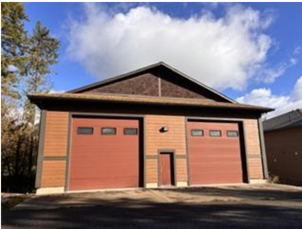
Roadside Elevation – Electric Overhead Doors 14'H x 14'W.
